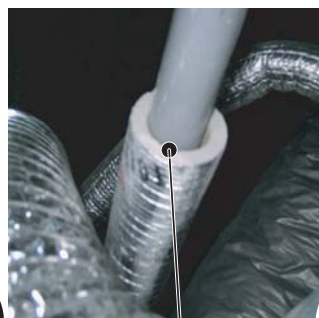
Fitting insulation
