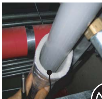
Loose fitting wrong insulation
