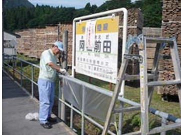
Painting guardrails at the Ani-Maeda Station
