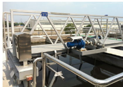
Reuse of wastewater for cooling water
