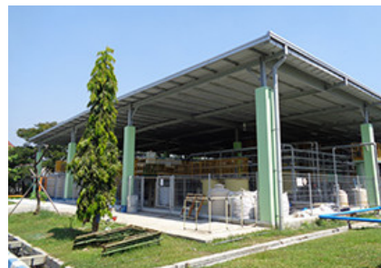
Wastewater treatment facility
