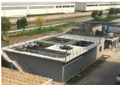
Wastewater treatment facility
