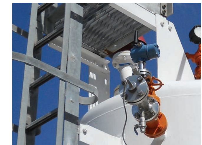
Rosemount 2160 installation
