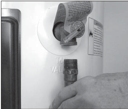
Figure 11 - Removing the T&P Relief Valve discharge pipe.
