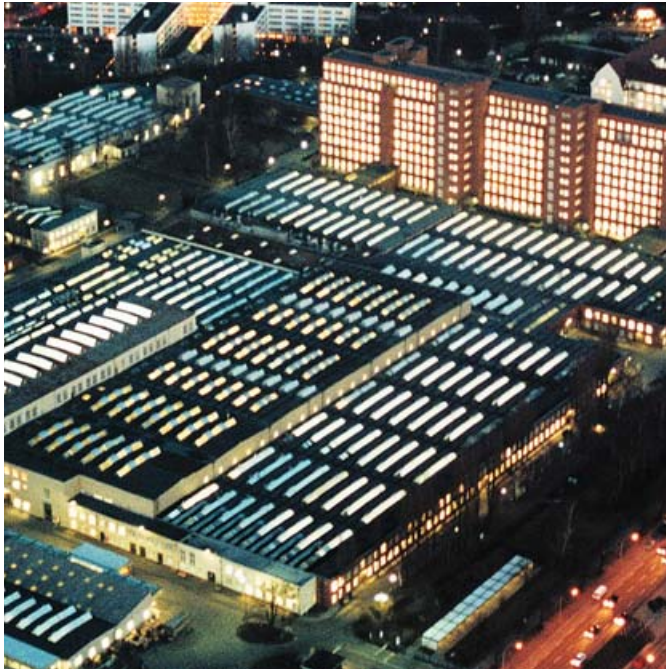
Switchgear Factory, Berlin
