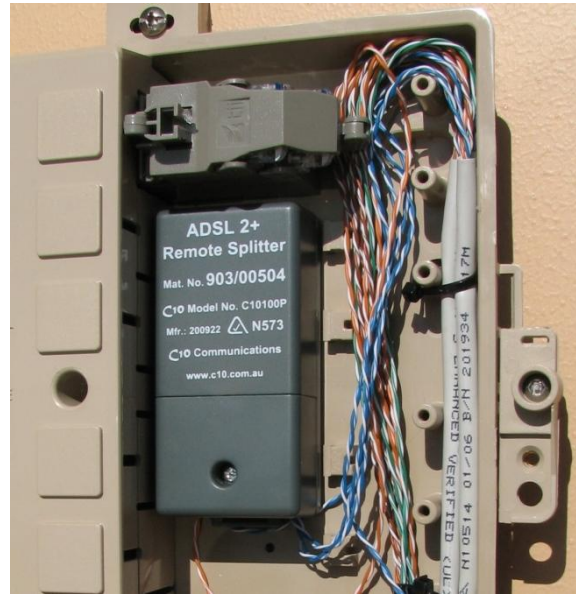
(b) Central filter in the customer side
