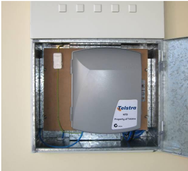
Figure 129 Telstra FTTP PSU with optional battery backup (obsolescent type)
