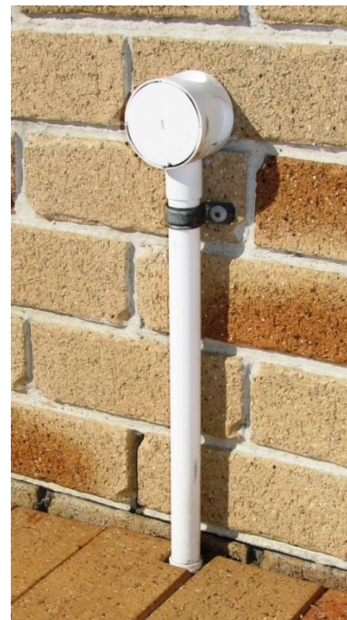
Figure 38 Sealed CAN (“AussieDuct”) junction box (obsolete)
