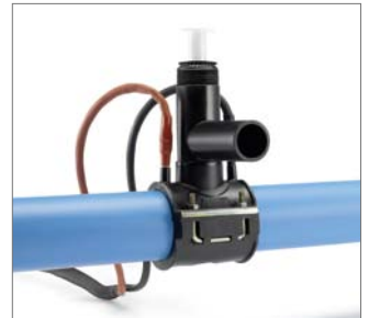
Fig. 59 7. An acoustic signal sounds once the welding process has been completed. The connections can then be removed.
