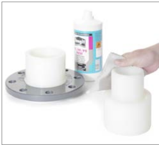
Fig. 117 Neither the flange nor the reducer are scraped prior to welding. Instead, both are merely cleaned.
