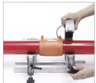
Fig. 106 At the conclusion of the "Cool: ... min." time indicated on the fitting, the universal pipe clamp can be removed.
