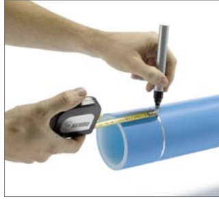
Fig. 40 2. Mark the scraping zone as illustrated in Table 8.
