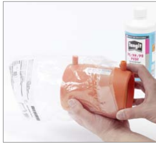
Fig. 96 Now remove the FUSAPEX electrofusion fitting from its bag. If necessary, clean the fitting with Tangit cleaner.
