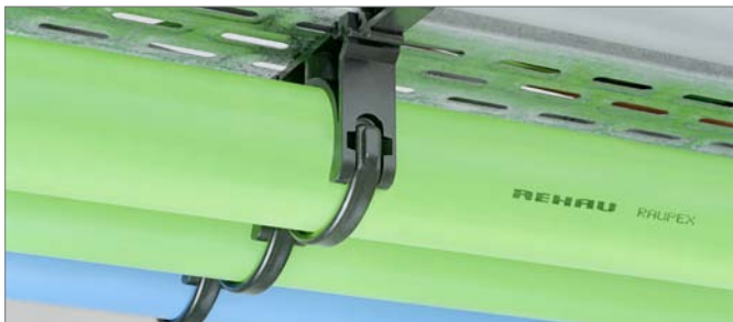
Fig. 131 RAUPEX pipe installed below or beside a cable carrier system
