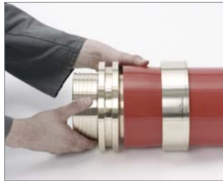
Fig. 30 5. Insert the fitting into the pipe. After a short time, the fitting will be firmly seated in the pipe (memory effect).
