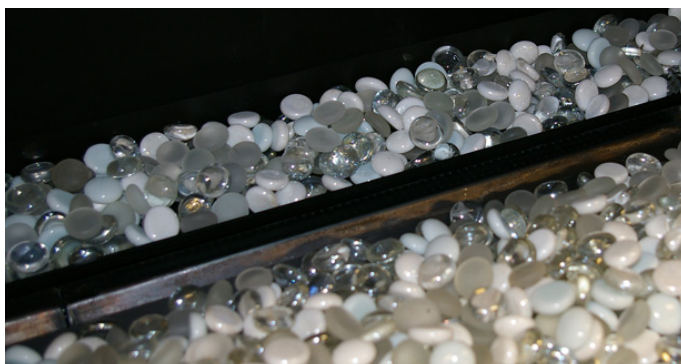
Figure 26. Completed firestone installation. Second Gen burner shown.
