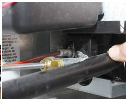
With the cover removed, inspect the burner and electrode assembly for rust or debris that may adversely affect performance.
