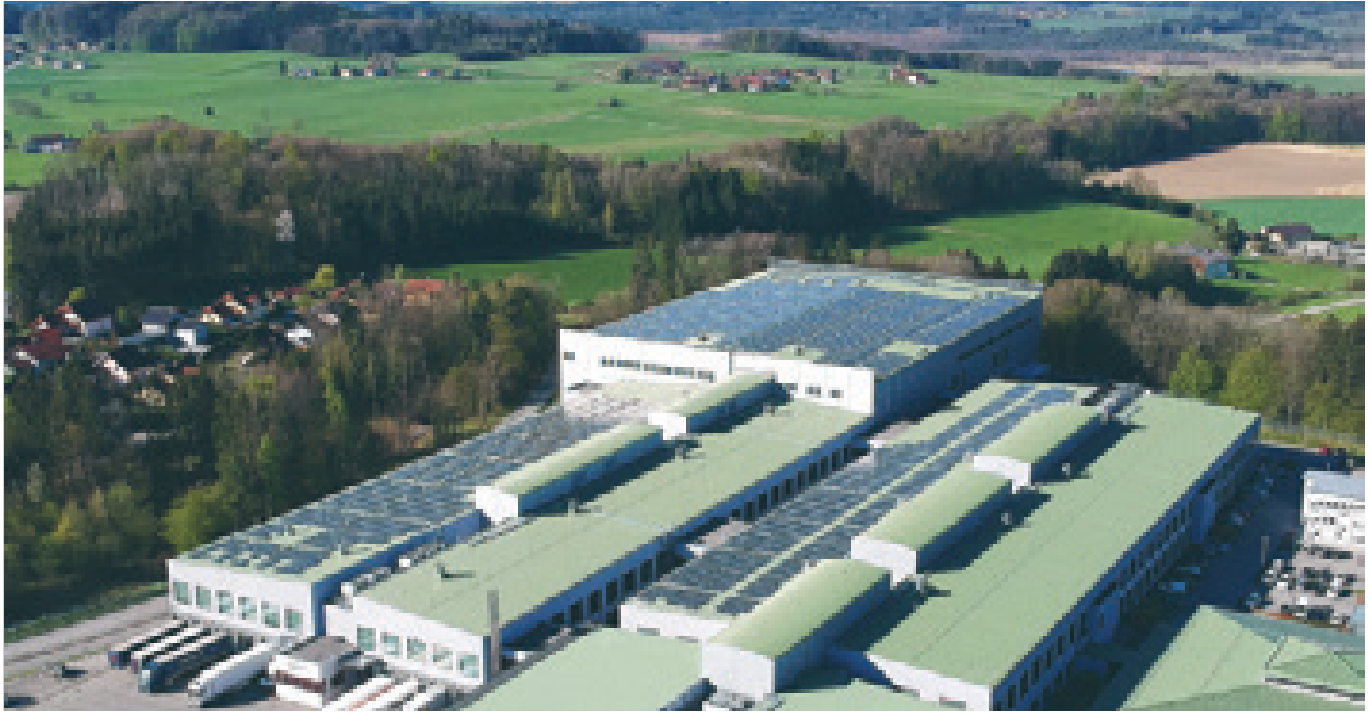
With a capacity of 1.5 megawatts, B&R's rooftop photovoltaic system is currently the largest self-consumption station in Austria.
