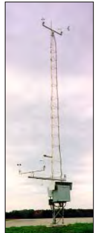
Weather Station with 30' Tower
