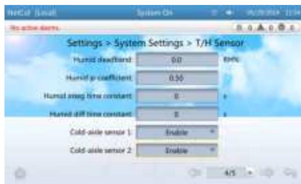
Figure 4-53 Enabling a humidity and temperature sensor
