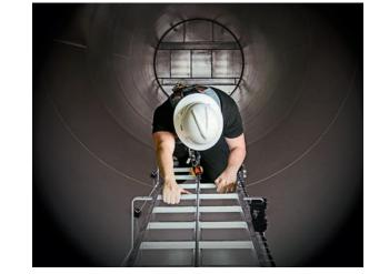
Allows for hands-free movement up and down the entire height of the fixed ladder, eliminating the need to disconnect and find new tie-off points.
