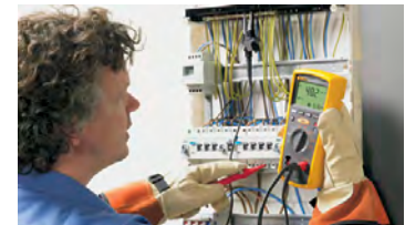
Insulation test at a distribution panel
