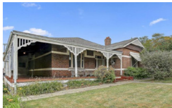
Figure 3 - Great Eastern Highway, Greenmount Source: CoreLogic
