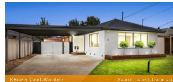
8 Broken Court, Werribee Source: realestate.com.au
