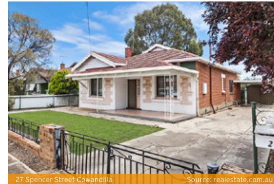
27 Spencer Street Cowandilla
