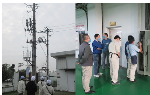
Electrical facilities audit in Vietnam
