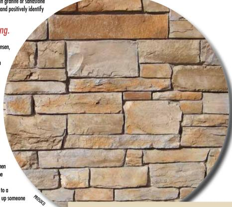
Natural or simulated? It's the job of this manufactured stone, a concrete product, to
