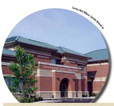
A typical example of today's masonry, the City Building, Edgewood, Ky., features brick, architectural block, precast concrete and manufactured stone. The rules for successful post-construction clean down of such buildings vary from procedures for cleaning buildings of mostly one type of masonry.
