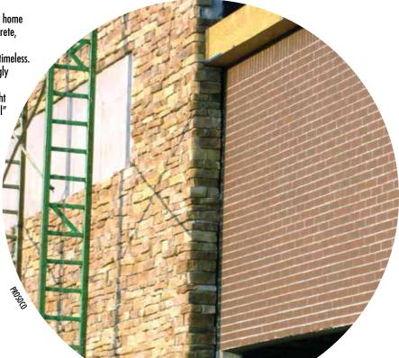
Manufactured stone and clay brick co-exist in this under-construction shopping mall in Olathe, Kan. Different masonry types in the same structure can make post-construction cleandown challenging.
