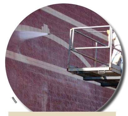
We're not talking garden hose here. Plenty of water, in both the pre-wetting and rinsing steps, is vital to a successful post-construction cleandown of new masonry.
