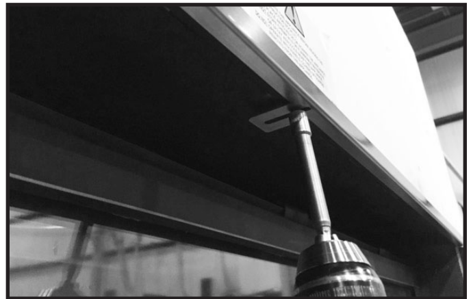
Figure 10.5 Install Trim Ring
