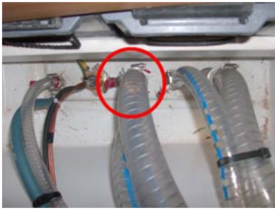
Drainage - Galley sink + Draining rack
