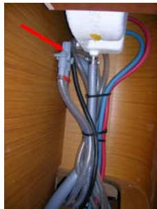
Anti-siphon valve (Reference 9)
