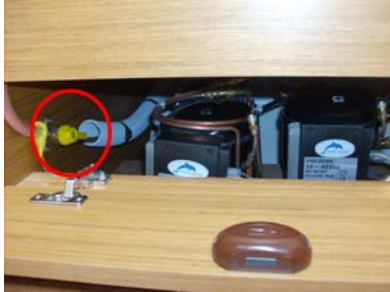
Opening valve / Reheating gas closing (Reference 1)
