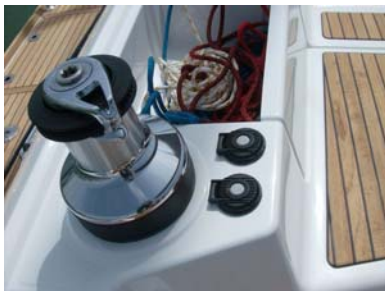
Electrical contactors - in the cockpit
