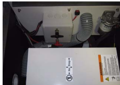
Anti-siphon valve (Reference 9)
