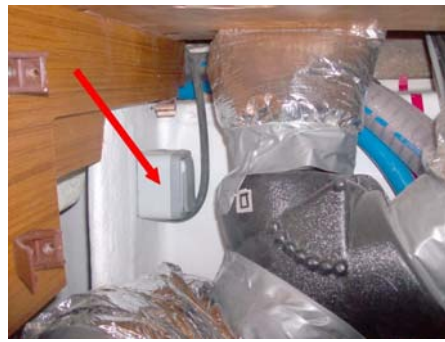
Supply valve - House water (Reference 3)
