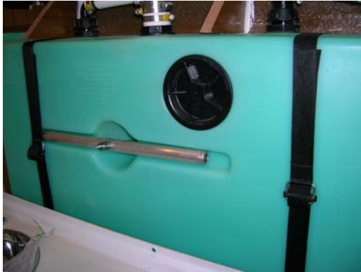
Detail - Tank Capacity: 80 litre Location: in each bathroom
