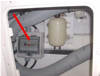
Breaker 220V 63A /32A - Port aft locker
