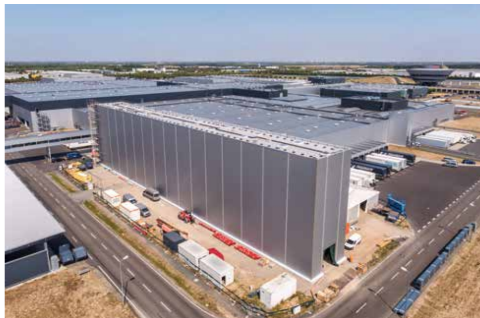
AUTOMATED SMALL-PARTS STORAGE SYSTEM
