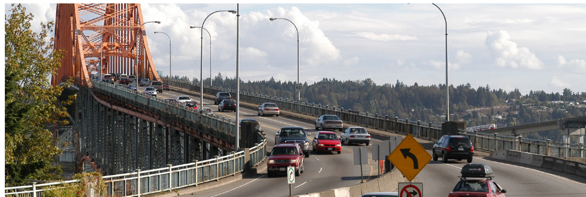
Photos of the existing Pattullo Bridge.
