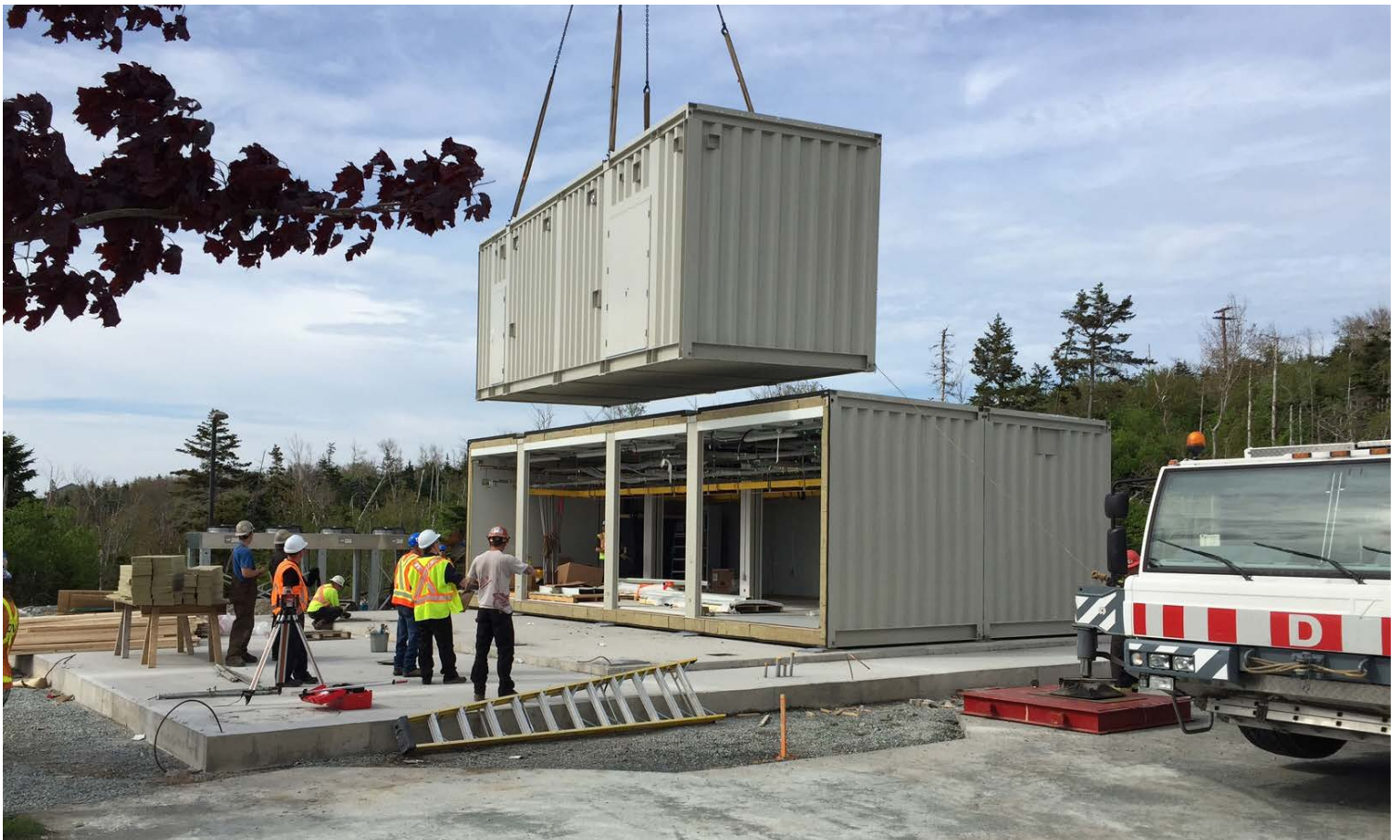
Installation of Vertiv™ SmartMod™
