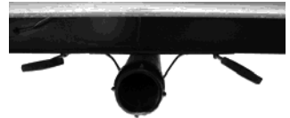
Fig 8.8 Black/Grey tank dump valves
