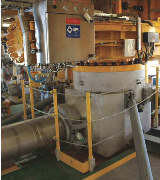
Emerson has provided four HIPPS top-entry API 15000 FCT valves with Biffi actuators for an offshore platform in the North Sea. (Photo courtesy of Emerson Automation Solutions)
