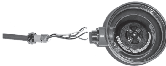
Figure 3-9: Installing the gland body
