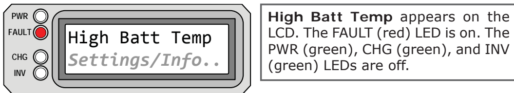
Figure 5-23, High Battery Temperature Fault
