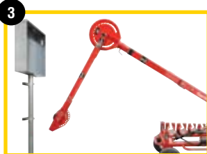
3 Align with conduit, properly adjust booms
