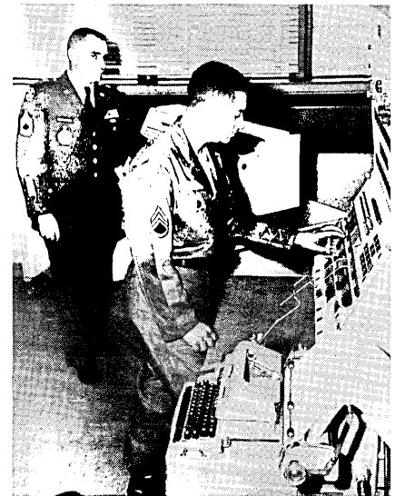
-- The student, foreground, is learning to operate MOBIDIC on the trainee console. The instructor, rear, monitors the problem at the master console. The flexowriter at the student's right prints out trainee's mistakes.
