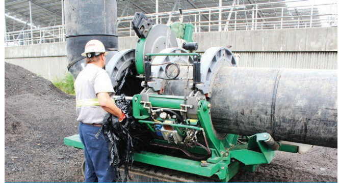
HDPE PIPE FUSION SERVICES
