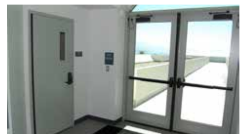
Top: Inside pushbutton on electronic lock allows door to be locked safely from inside, yet occupants can exit without restriction.
