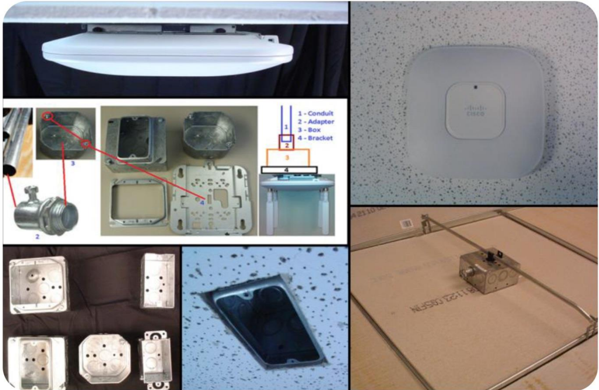
Figure 25. Mounting an access point onto an electrical conduit box (ceiling T-bar or conduit)
