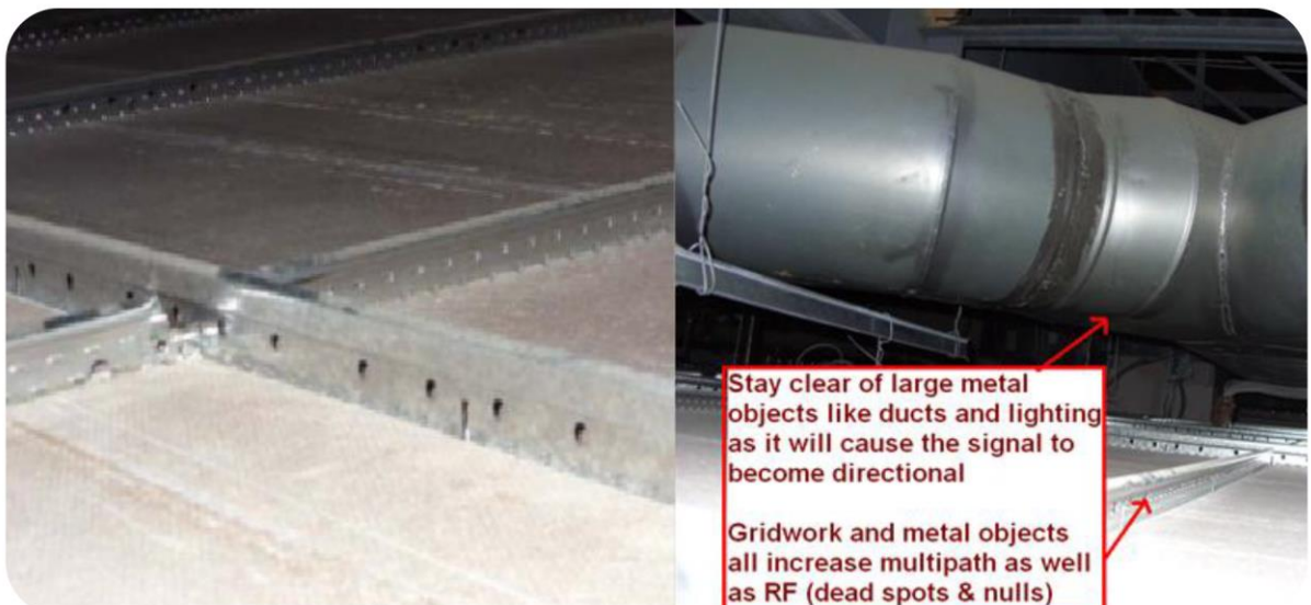
Figure 21. Installing an access point above ceiling tiles: Pick an area clear of obstructions, and avoid ceiling clutter
