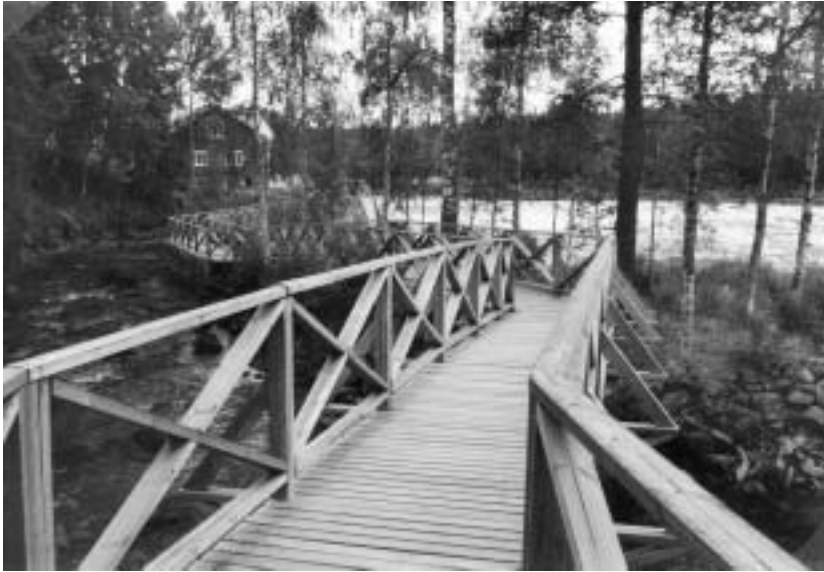
Fig 6.6:1 A good bridge construction
