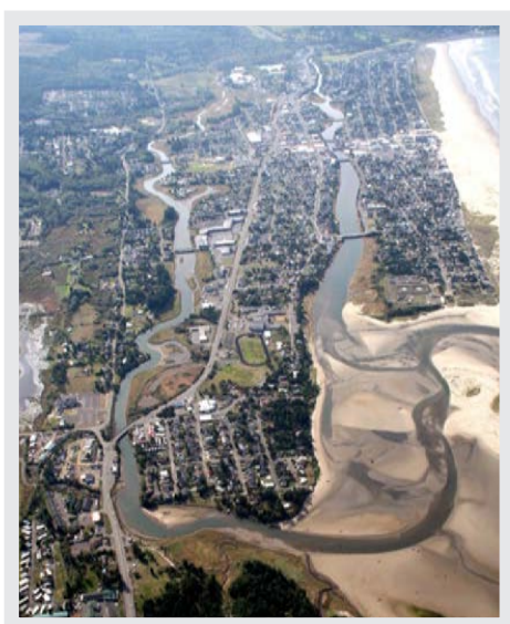
Tsunami Vulnerability: City of Seaside with 83% of its population, 89% of its employees and almost 100% of its critical facilities in the tsunami inundation zone. Source: Horning Geosciences
