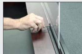
Step 3 - Secure with included set screws
