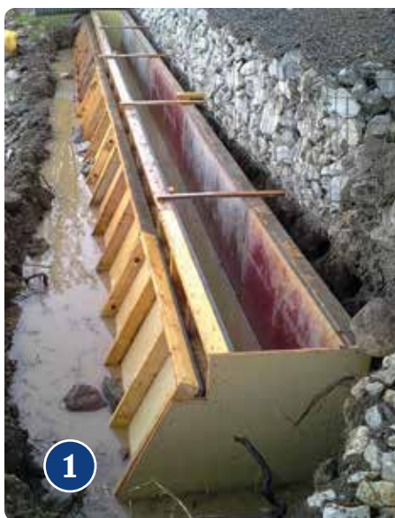
1) Concrete footing for stacked decorative block wall formed and ready to pour.
