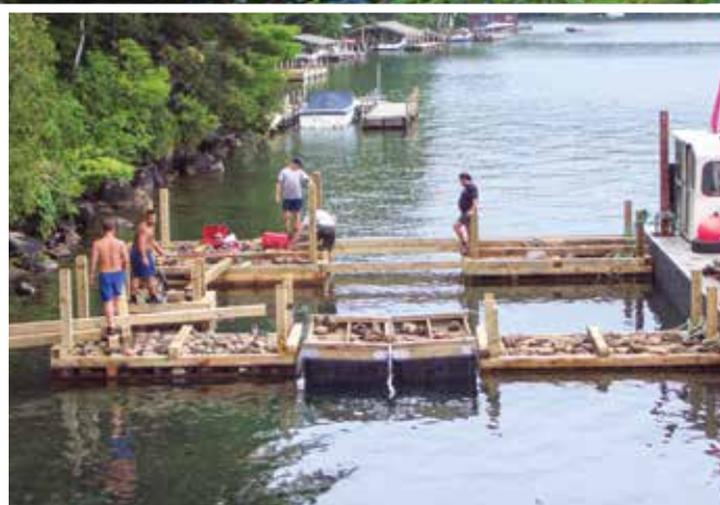
Crib dock in progress.
