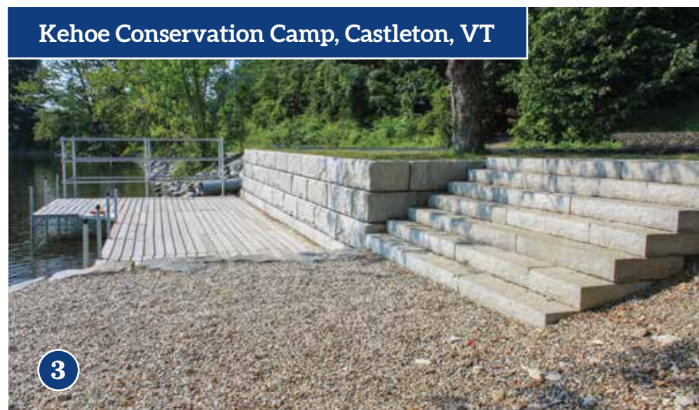
3) Project complete with stacked block wall, concrete steps and our seasonal dock system.
