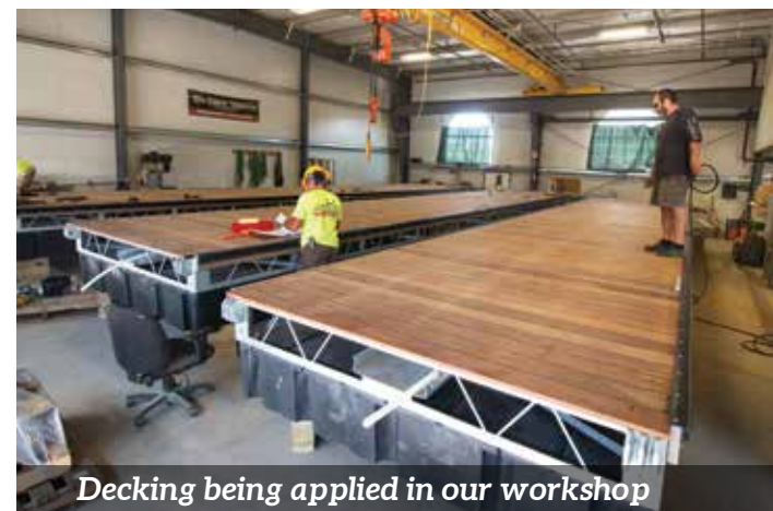
Manufacturing of the dock frame
