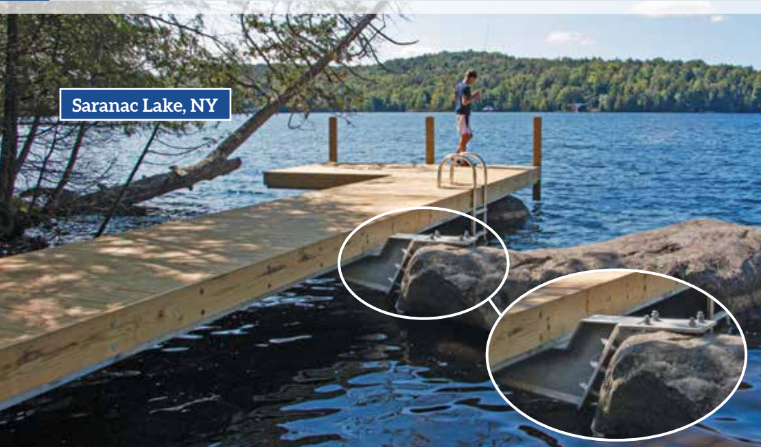
Cantilevered end of dock mounted to boulder with custom mount.
