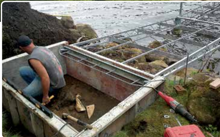
Above Bottom: A concrete pad is being formed to serve as the shore hitch for the above articulating dock.
