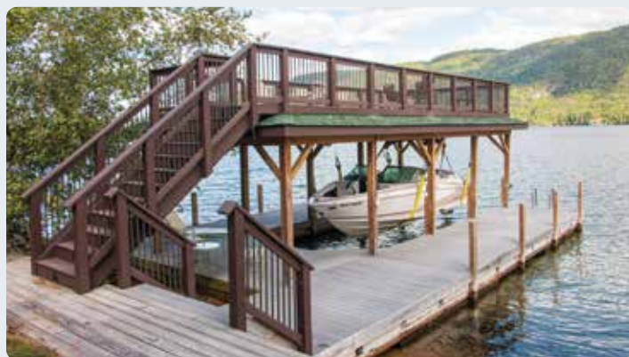
Crib dock with sundeck style boathouse and sling style boathouse lift.
