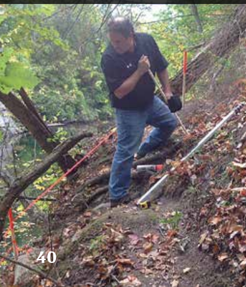
Measuring for a new stair system.
