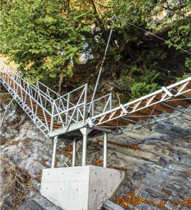
Freespan stairs with lower section that raises for winter storage.
