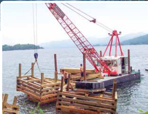
New cribs being moved into position.
