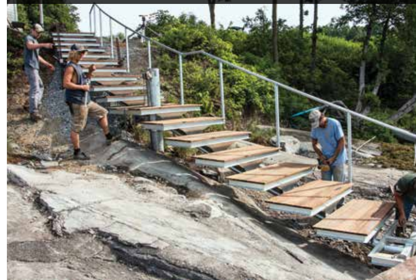
Curved mono-beam stairway during installation
