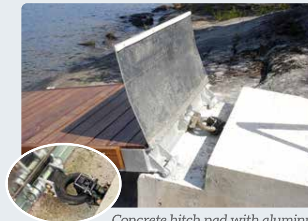
Concrete hitch pad with aluminum tread plate and pintle hitch.
