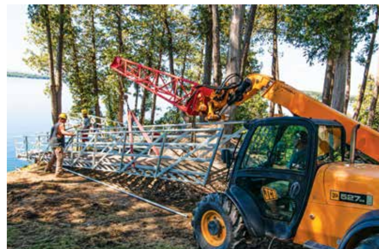
Stairs being installed.
