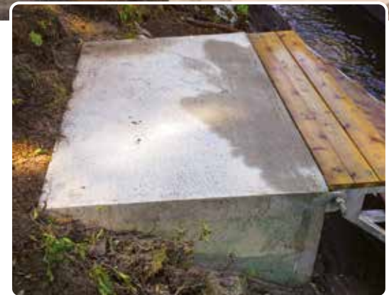
Above & Right: "L-shaped" articulating dock with cedar decking. A concrete pad serves as a shore hitch.
