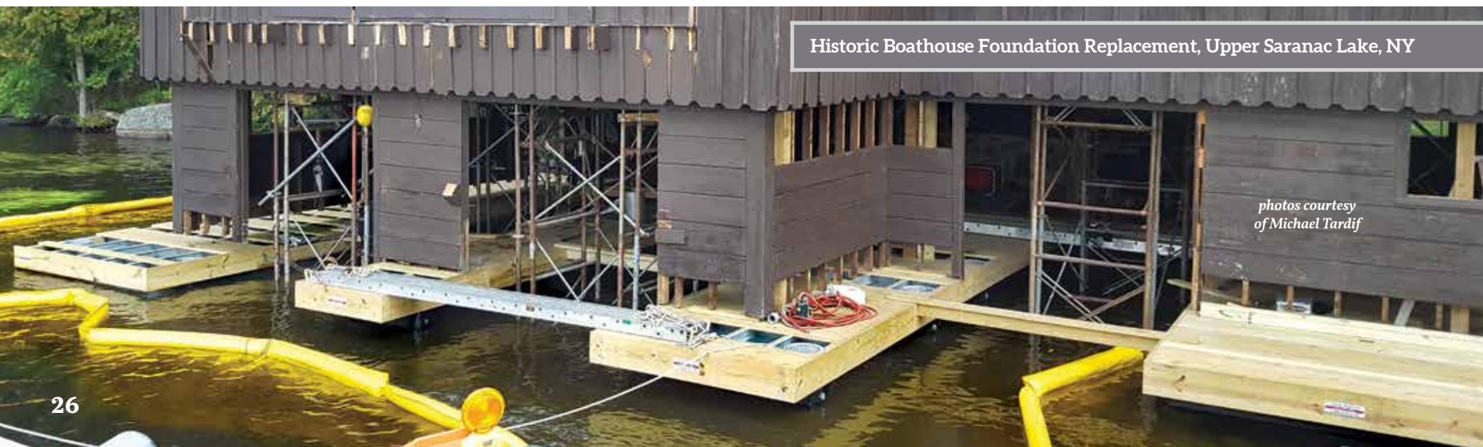
Piles being placed for the new pile dock foundation.
