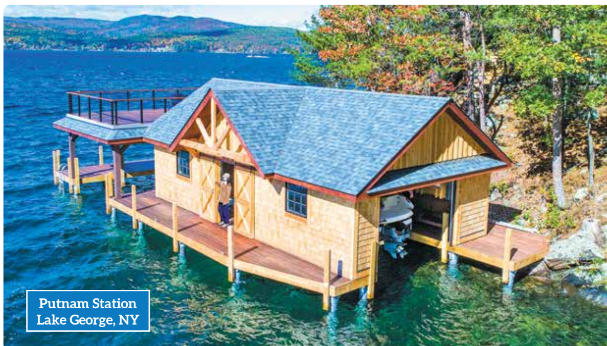
Land-based pile dock foundation with boathouse designed & built by The Dock Doctors.
