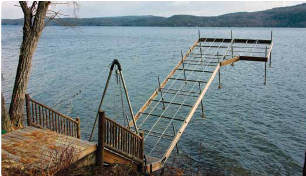
Above & Right: "L-shaped" articulating dock with cedar decking. A concrete pad serves as a shore hitch.
