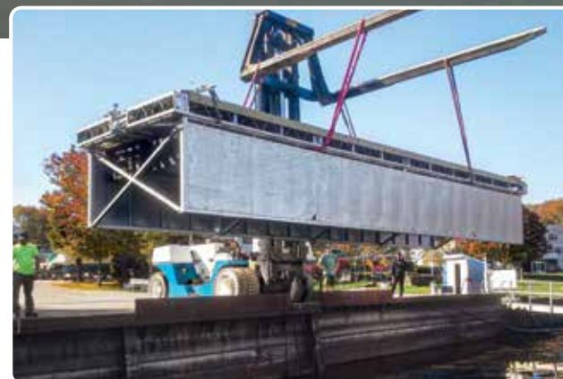
Wave attenuator being installed.
