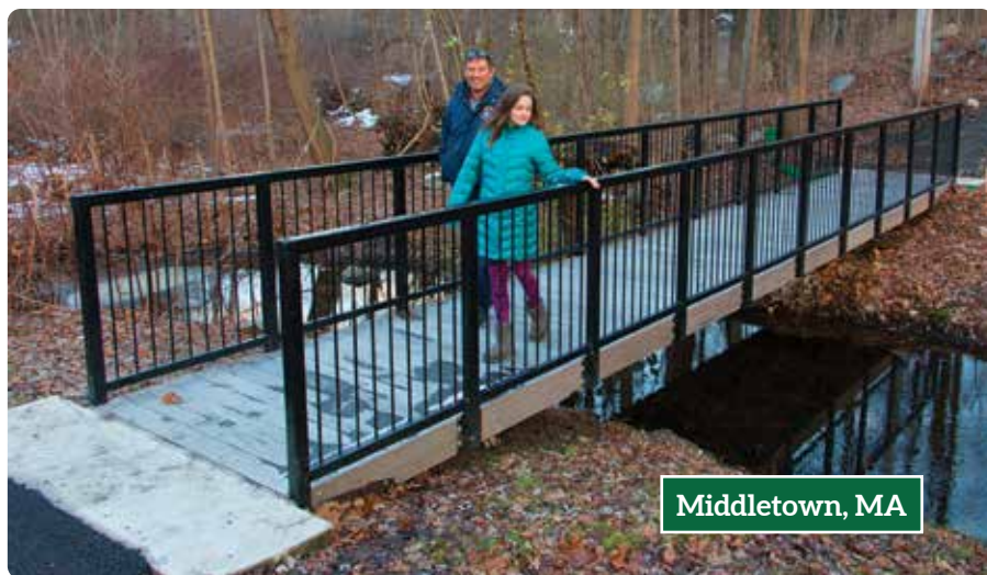
Pedestrian bridge with black powder coated railings.
