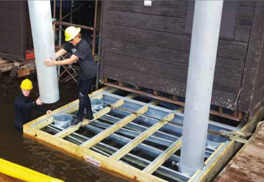
Piles being placed for the new pile dock foundation.
