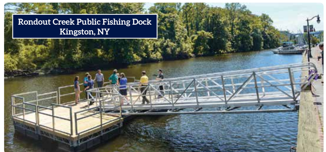
ADA accessible gangway.
