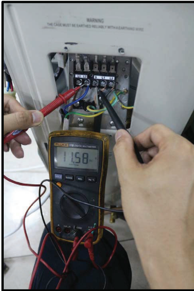
Fig. 31 — Test the DC voltage
