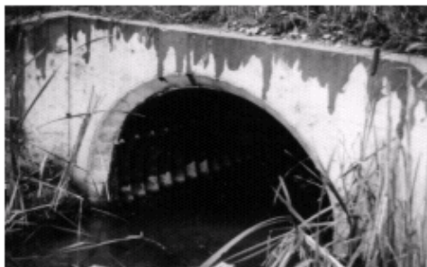
Head wall with beveled edge inlet
