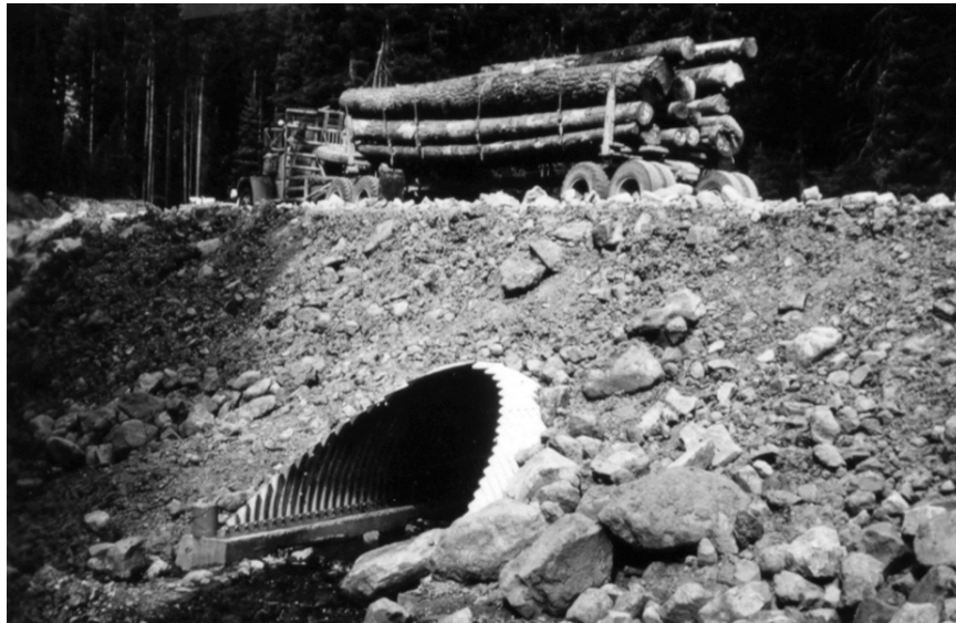
Figure 9.22 Culvert on Spread Footings to Retain Streambed for Fish Passage
