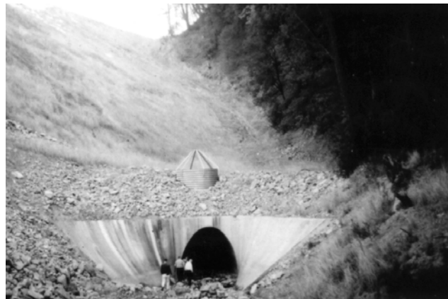
Figure 9.24 Vertical Riser for Relief
