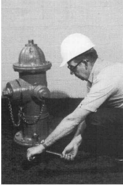
1. Loosen Nuts on Safety Flange Bolts.
