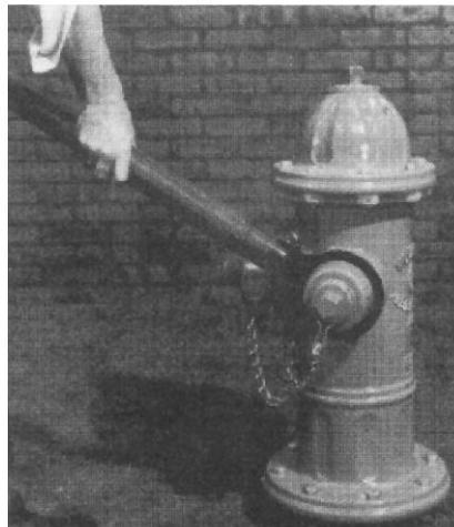
5. Thread new Nozzle into Upper Barrel, attach A-316 Nozzle Wrench as described in Step 3, and tighten Nozzle to approximately 600 ft-lbs torque (100 lbs. pull on a 6' lever).
