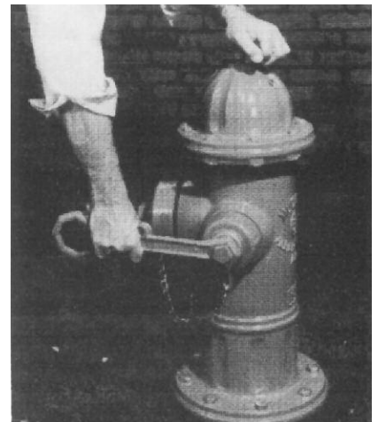
7. Replace and tighten Nozzle Cap.
