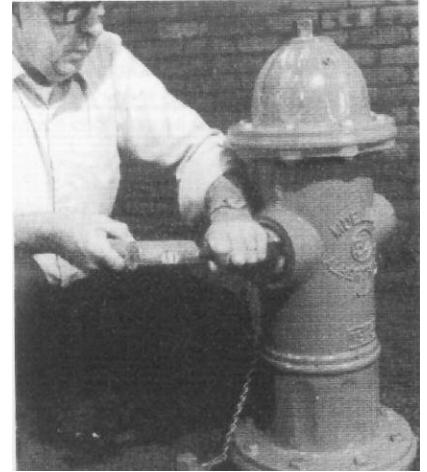
6. Remove Nozzle Cap and A-316 Nozzle Wrench. Place the Nozzle Lock (Part 143137), lengthwise in the slot formed by either of the Nozzle Drive Lugs and the Barrel Bore. Drive the Nozzle Lock in place by striking the Nozzle Lock Installation Tool (Part 143132) several times with a heavy brass hammer.
