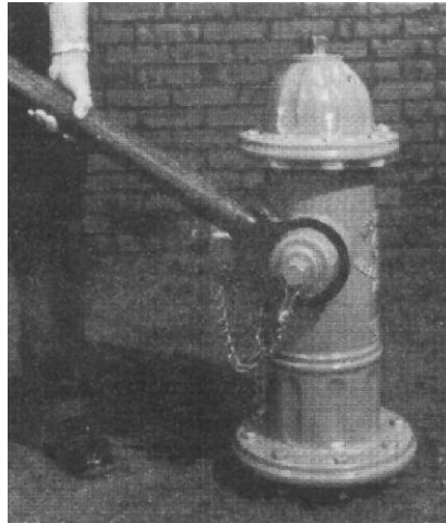
4. Remove Nozzle. The Nozzle Wrench may be struck with a heavy brass hammer or additional leverage may be obtained by placing a length of 2" schedule 40 steel pipe over the handle of the Nozzle Wrench.
