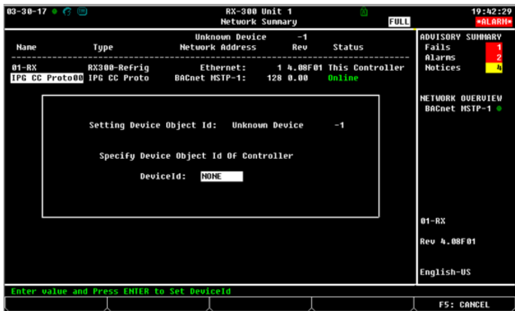
Figure 14-6 - Commissioning the BACnet Device
