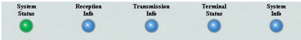
Figure 45: System Control Center button links
