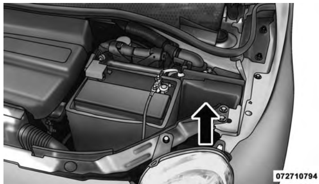
Front Distribution Unit
