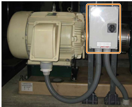
Figure 6-11 Example: Device for removal of power for prevention of unexpected start-up
