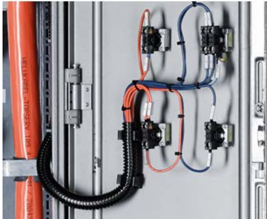
Figure 6-70 Example: Installation in doors with flexible cables
