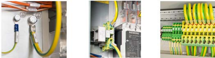
Figure 6-45 Examples: Components of the protective bonding circuit
