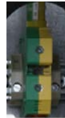
Symbol IEC 60417-5019 Marking by the letters PE Identification by the bicolor combination GREEN-AND-YELLOW
