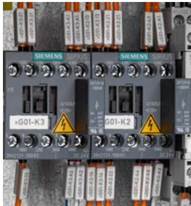
Figure 6-22 Labeling of components that are still live even though the supply disconnecting device is open
