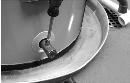
Figure 10 - Draining the old water heater.
