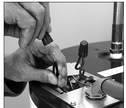
Figure 19 - Connecting the electrical wires.
