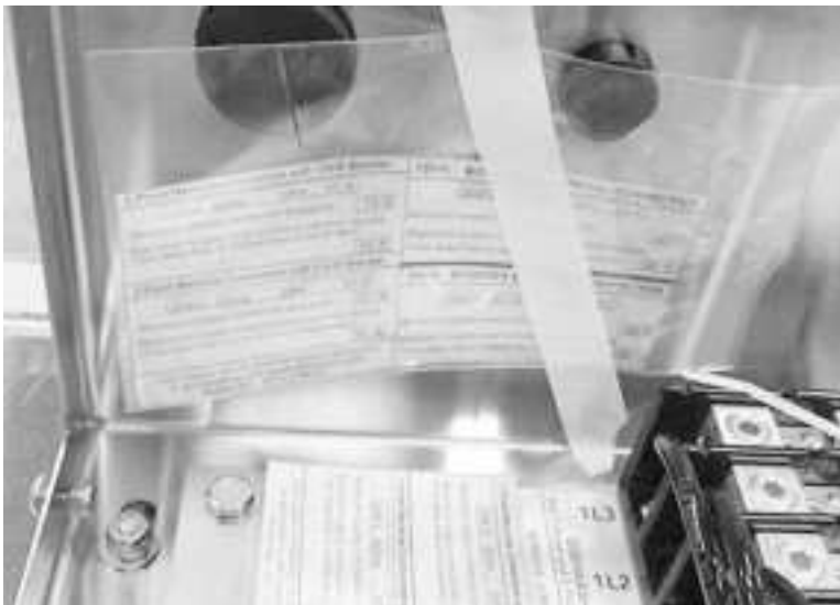
Fig.15 - The 2-point data plate is located in a plastic bag next to the terminal block.
