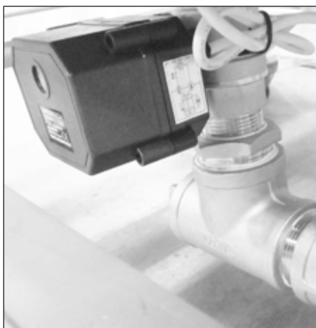
Fig. 6B - Electric Drain Valve
