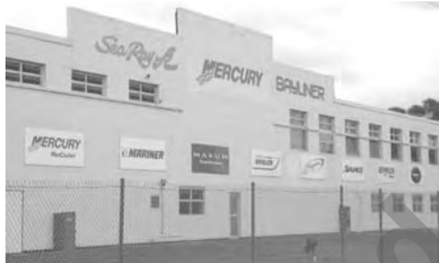
Figure 14:7 Un-reinforced masonry (besser block) construction
