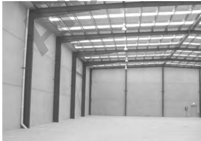
Figure 14:8 Concrete tilt-up construction
