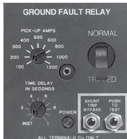
Ground Fault Relay
