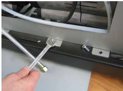
Fig. 9-12 – unscrew bolts from compressors
