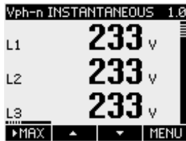
Figure 3-2 Display of the measured voltage in the case of connection type 3P4W
