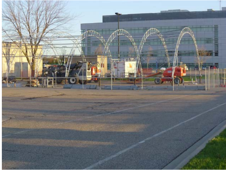
Figure 4-2: Initial Construction of Temporary Structure
